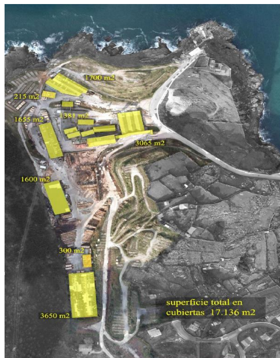
Figure 8: Potential roof area for PVT installation in Lekeitio [Barrizar 2017b].
