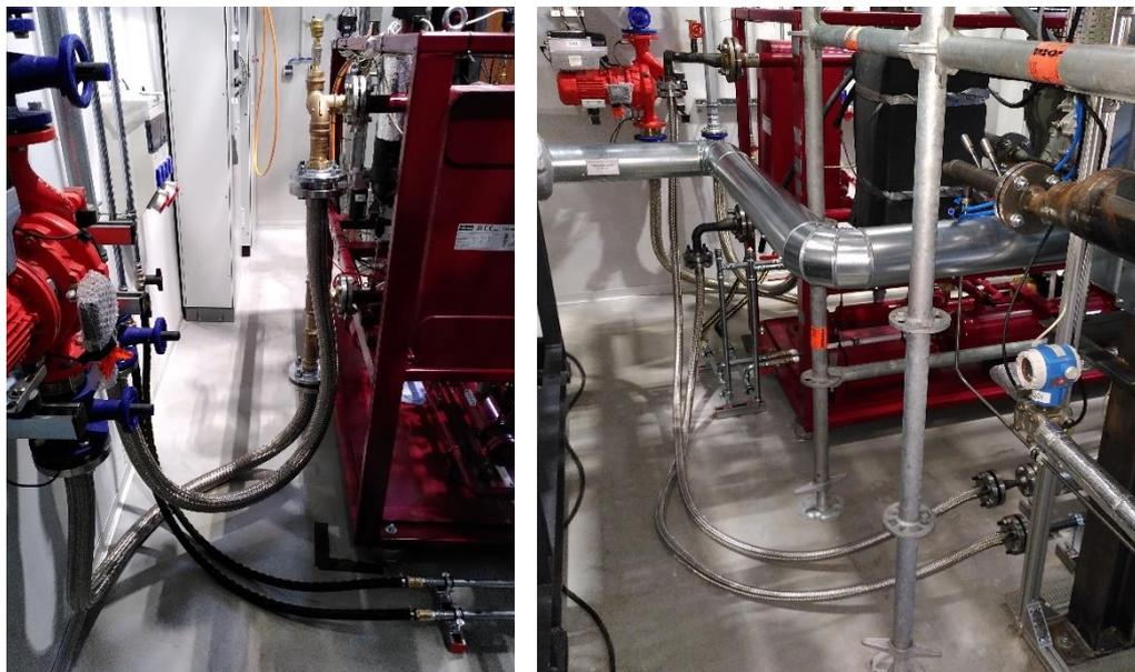
*Figure 23: ORC – Hose connections between condenser, expander cooling, subcooler and CWDN (left) and between preheater and SH-TESS water circuit (right)*
