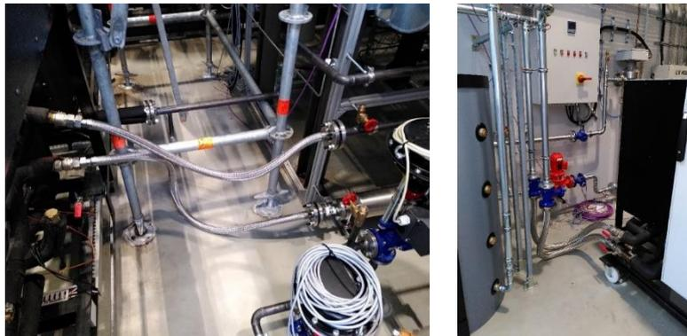
Figure 28: HTHP connections. Hose connection between HTHP and SH-TESS loop (left). Hose connection between HTHP and heat source (right)
