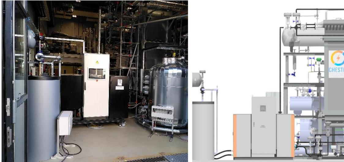
Figure 19: HTHP integrated into the laboratory CHEST system. Final arrangement (left) and 3D-drawing for planning system layout and pipe connections (right)
