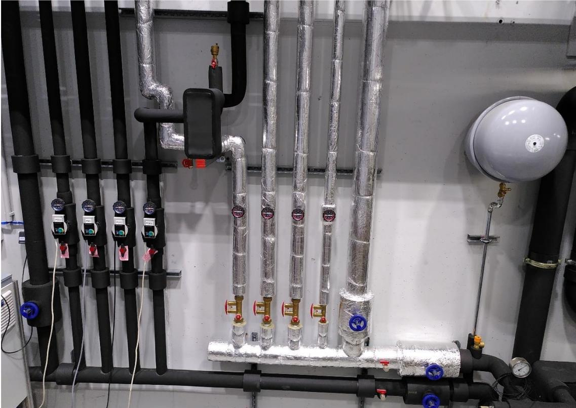
Figure 11: Setup of cooling water distribution from the CWN in the laboratory
