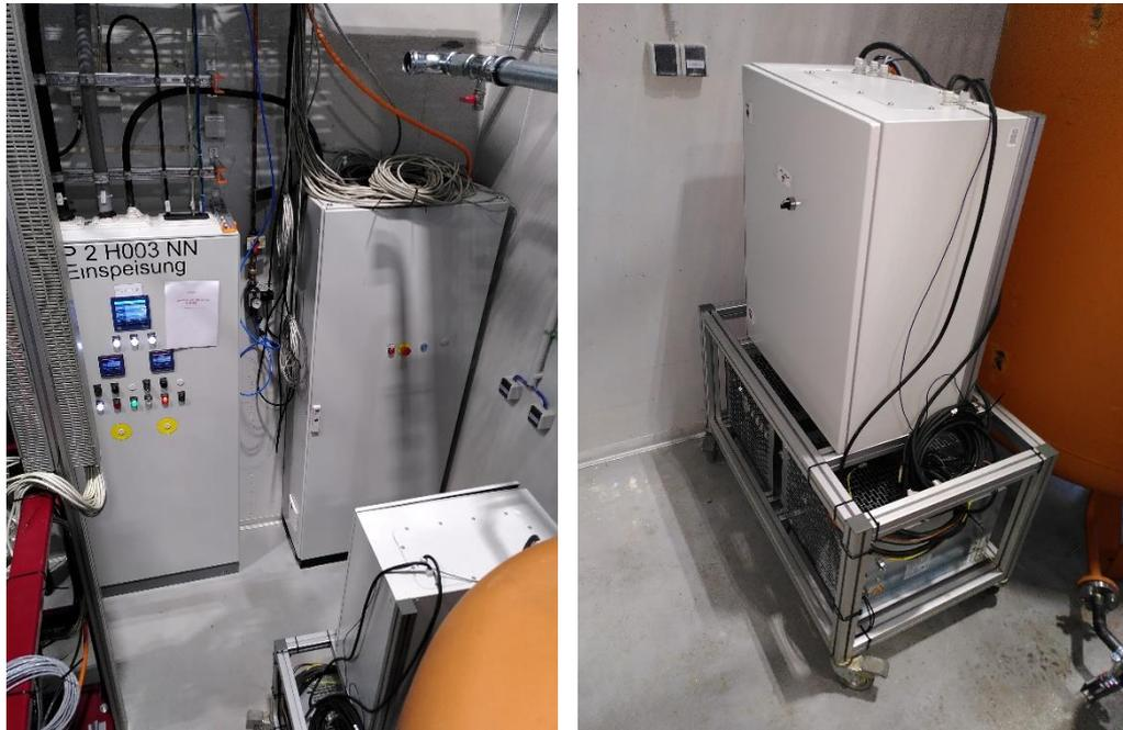
Figure 25: ORC – Feed-in point (left), control cabinet (left) and chopper cabinet (right)
