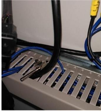
Figure 27: HTHP – loose parts in the control/power cabinet.
